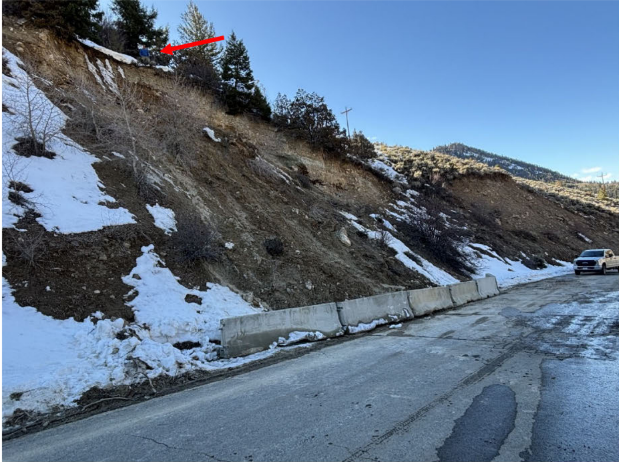
Figure 3 – A northwest facing view of the recent landslide taken shortly after the initial slide prior to this site visit. There is a person in a blue jacket at the top of the slide, marked by an arrow, for scale. The head scarp is approximately 10-20 feet tall. Some cobbles and boulders are seen sliding down the slope. Photo by T. Kummer (USBR) – 3/17/2025
