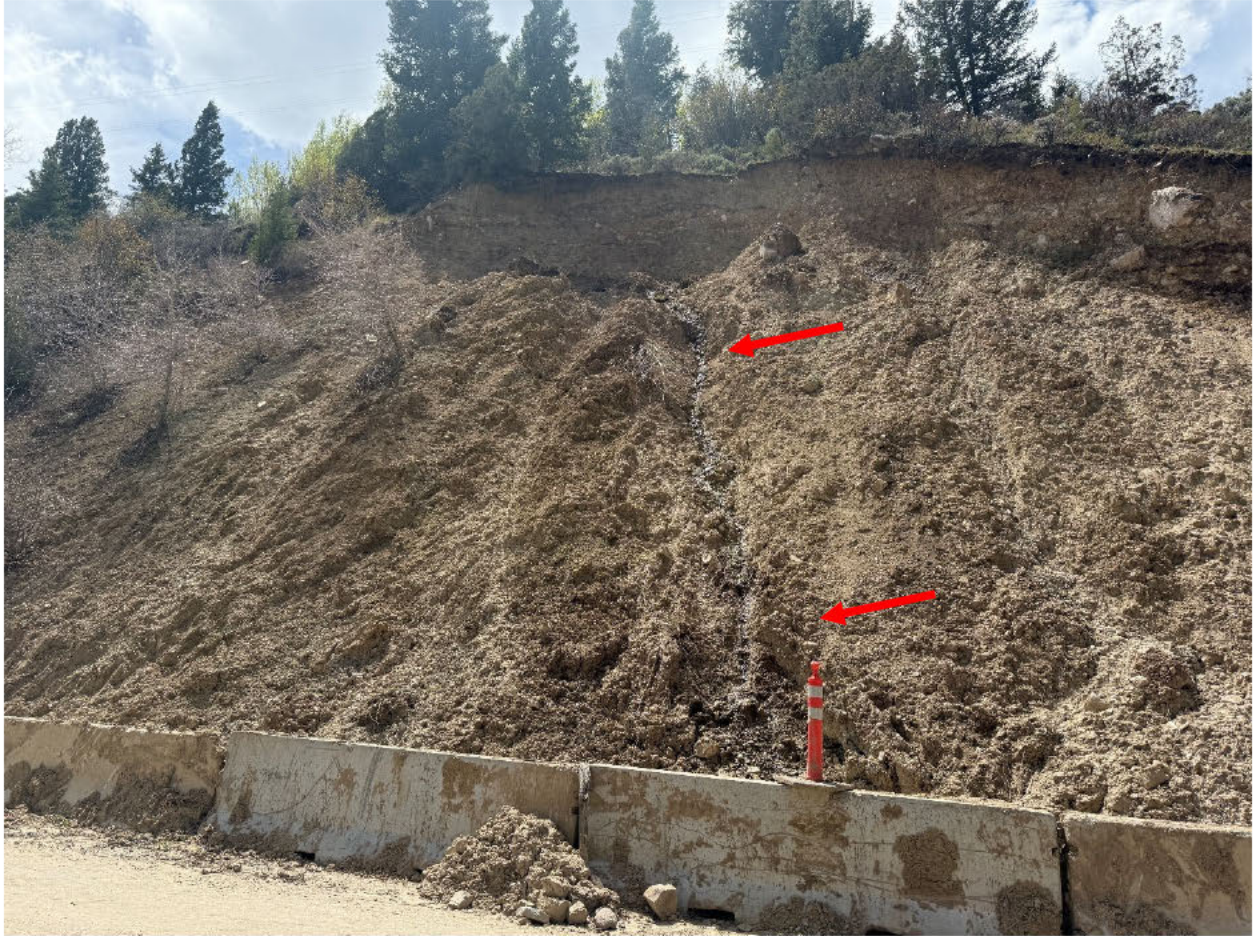
Figure 5 – A photo of groundwater exiting from the slide face seen during our site visit. The water exiting the slide is creating an erosional channel and saturating slide deposits towards the toe. The amount of water seen during our visit was minor compared to the amount of water seen exiting the slope following the larger slide events in March and April.
