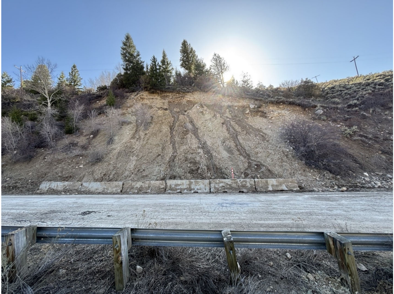
Figure 4 – A west facing view of the landslide taken prior to this site visit. Groundwater is seen exiting the slide in multiple areas along a similar plane. This plane is evidence of perched water tables bound by an impermeable layer of rock or soil.
